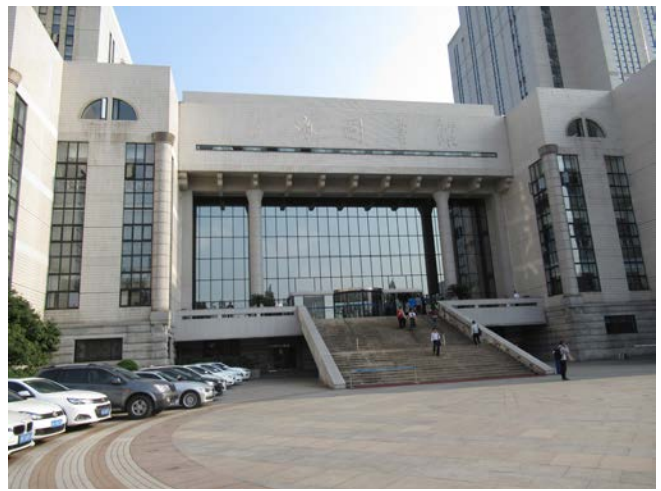
The Shanghai Library main building: entrance and maquette.
